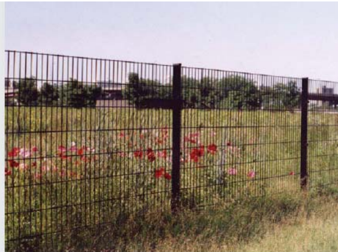
Double wire fence
